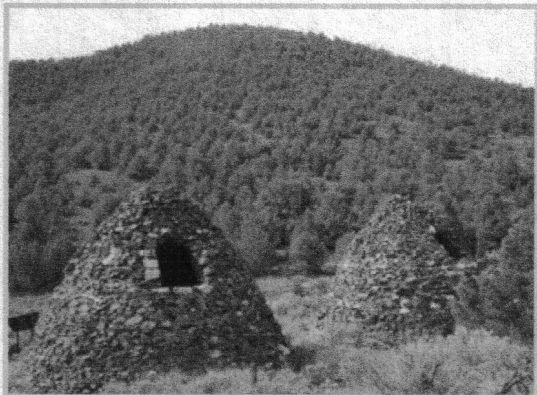
Two Charcoal Kilns just above the Old Ghost Town of Tybo. Built from local stone.
