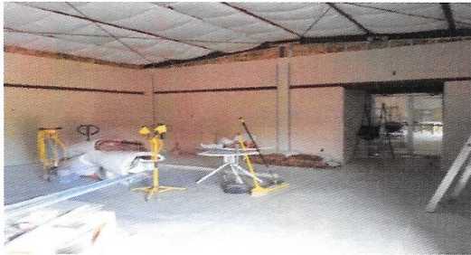
And the drywall is finished!
