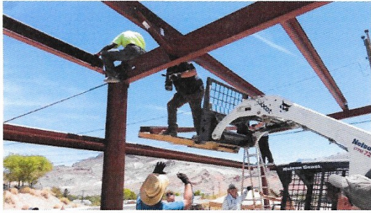
The last beam going up!
