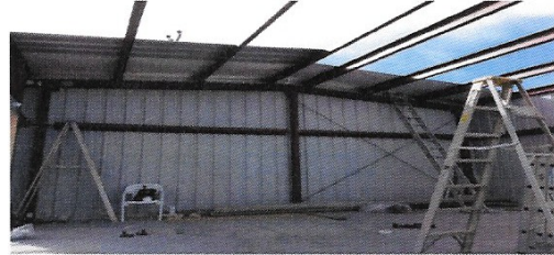
Putting the roof on!
