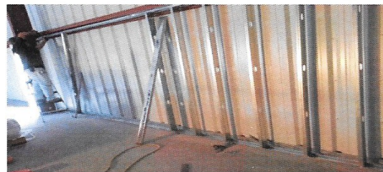
Ed Trumble framing in the walls
