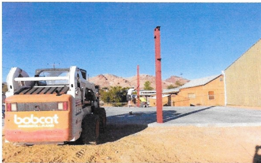
First Beams Going Up w/ Ken Nelson Construction
