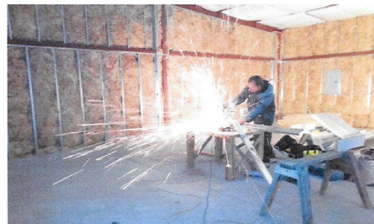
Ed Trumble cutting metal studs to frame walls!
